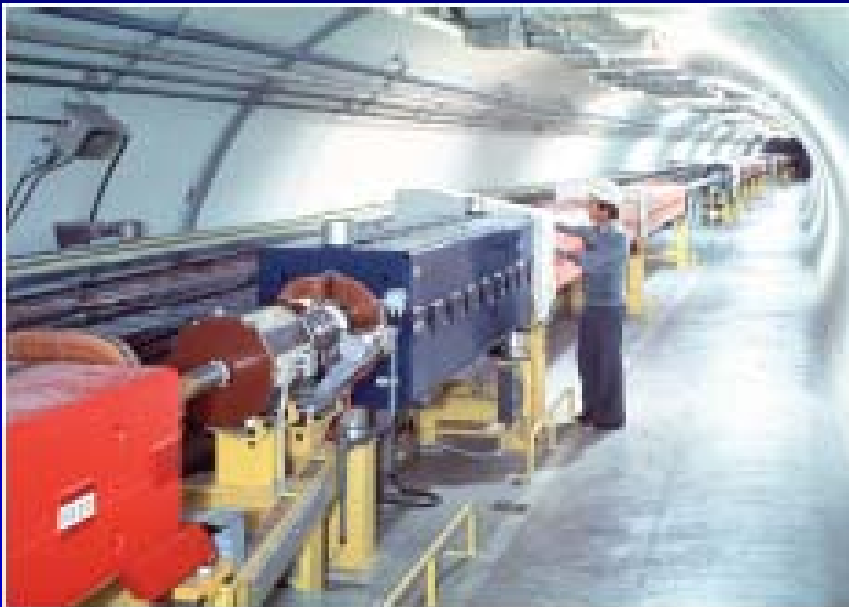
LEP Tunnel, 27 Km circumference
